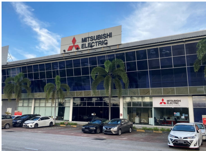
Mitsubishi Electric Sales Malaysia Sdn. Bhd., home of new Malaysia FA Center
