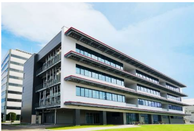
Net Zero Energy Test Facility “SUSTIE”
