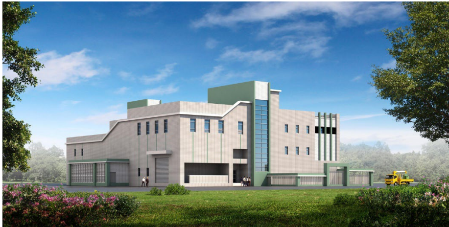
Rendition of substation where Taiwan's first STATCOM will be installed
